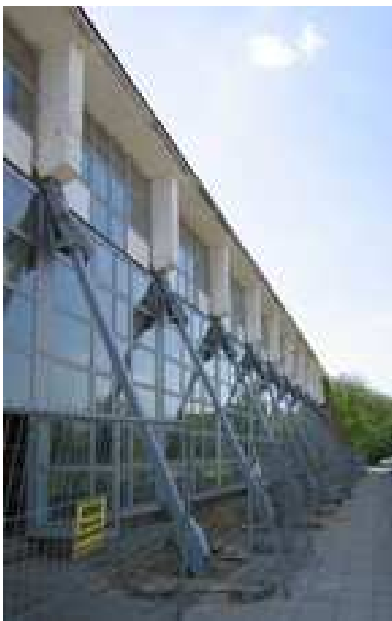
Fig. 11. The restored column line.
