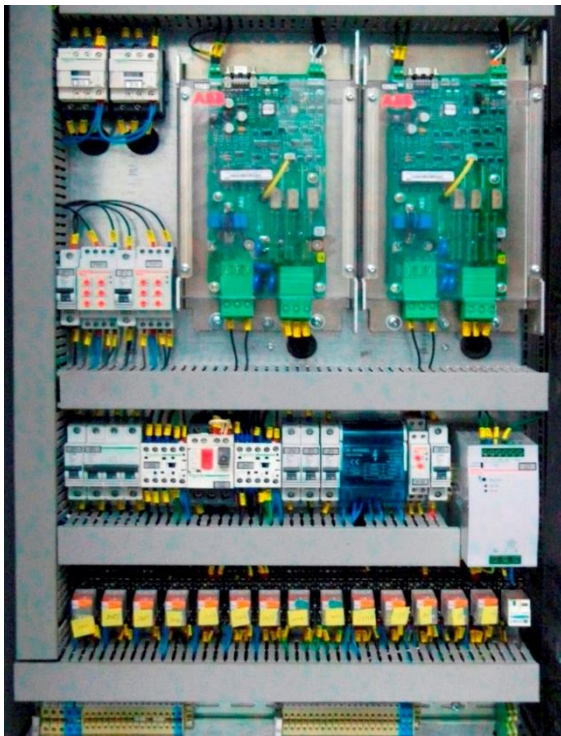
Fig. 13. Interior of the field circuits power supply cubicle with the FEX4 boards
