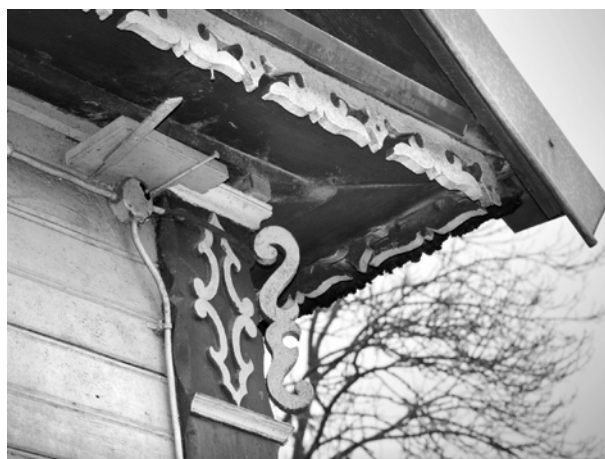
Fig. 5. Wood plank ornamentation of a cornice; photo by the authors, 2018
