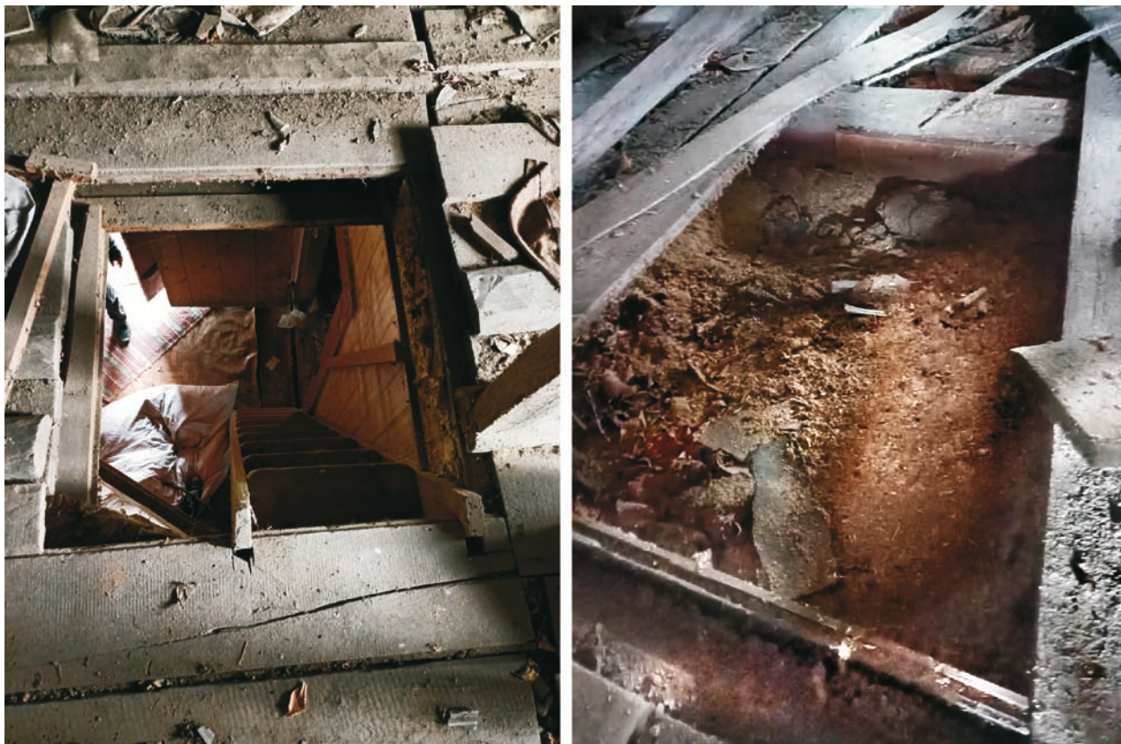
Fig. 11. Garret floor construction (a – ladder descending to the entrance hall; b – earthen insulation); source: the authors, 2021
