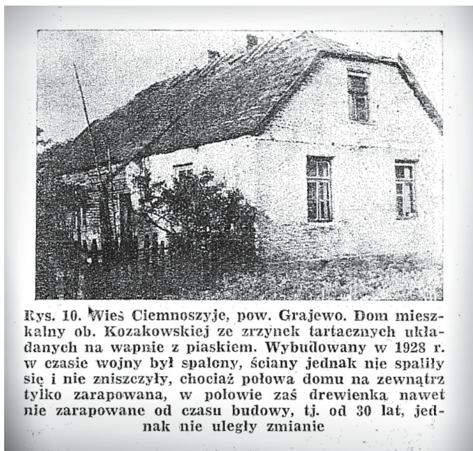
Fig. 2. A farmhouse made with cordwood in 1928 in Ciemnoszyje; source: M. Łukaszewicz [1958, p. 14]
