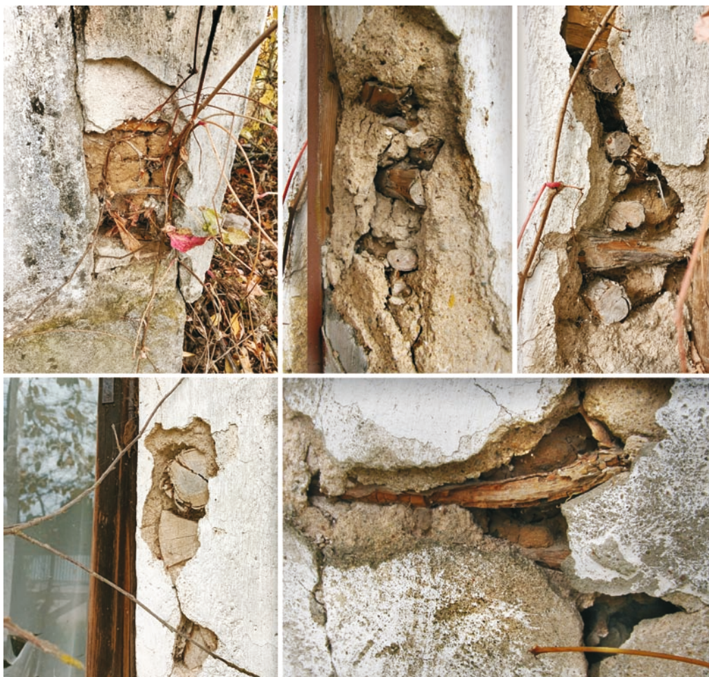
Fig. 4. A stone foundation of the house in Olszewo, its ornated plaster and two ceramic tubes for wooden floor ventilation; source: the authors, 2021
