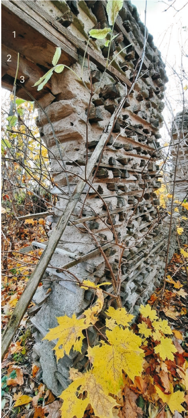
Fig. 10. Wall and carpentry details of the cordwood house in Rydzewo Kolonia: (1) door lintel; (2) door header; (3) mortise; photo: Renata Adamska and Katarzyna Karwowska, 2021
