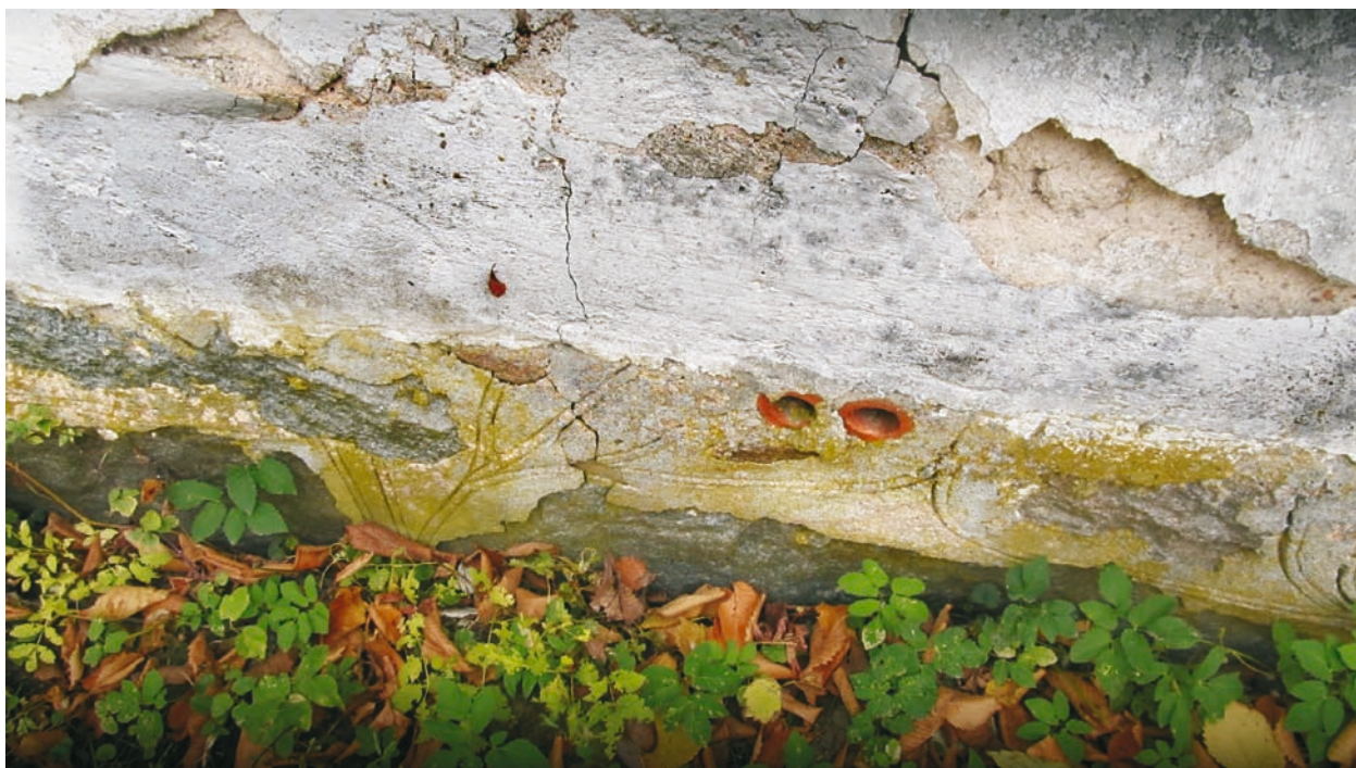
Fig. 4. A stone foundation of the house in Olszewo, its ornated plaster and two ceramic tubes for wooden floor ventilation; source: the authors, 2021
