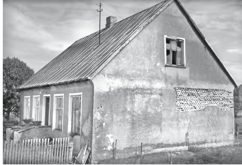
Fig. 11. A farmhouse made with cordwood in Pierńczykowo; photo: the authors, 2018
