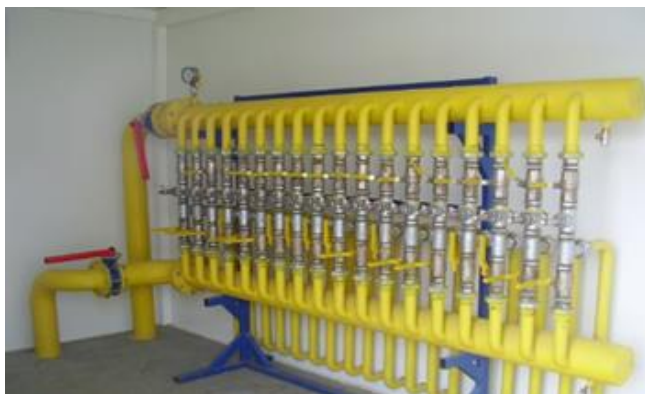
Fig. 3. Connection of gas wells to main pipelines (13)
