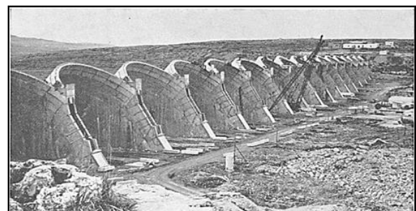
Fig. 2. El Mefrouch multi-arch dam [26]
