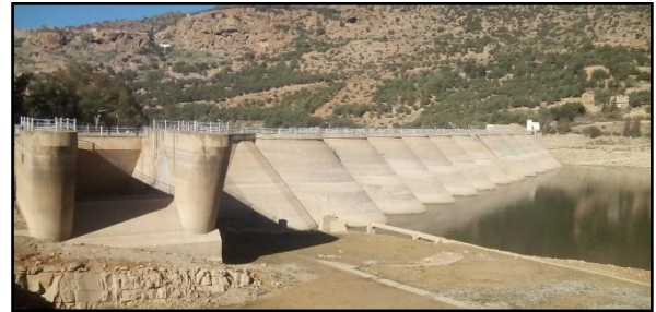
Fig. 1. Beni Bahdel multi-arch dam [27]
