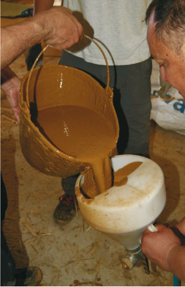
Fig. 36. The right consistence of clay-water mix, 2021; photo by the author
