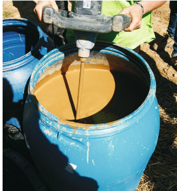
Fig. 34. Making of clay--water mix, 2021; photo by the author
