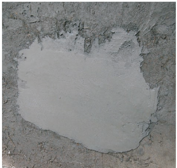
Fig. 39. A finer plaster layer has been plastered onto a coarser layer. Still the finer layer can be worked even finer. This is "blue clay" in Norway, 2014; photo by the author
