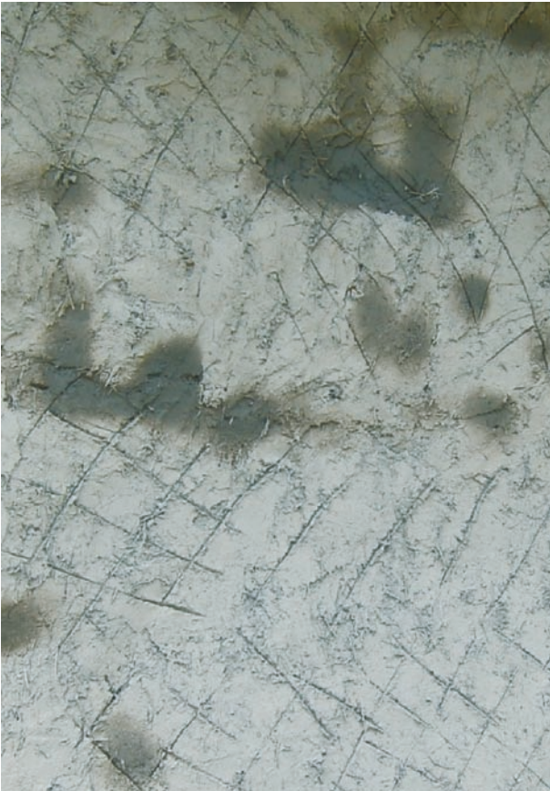
Fig. 32. Clay based mortar on a straw bale house. The mortar is naturally coarse and intentional cut marks have been made to make the coming plaster layer stick better, 2015; photo by the author
