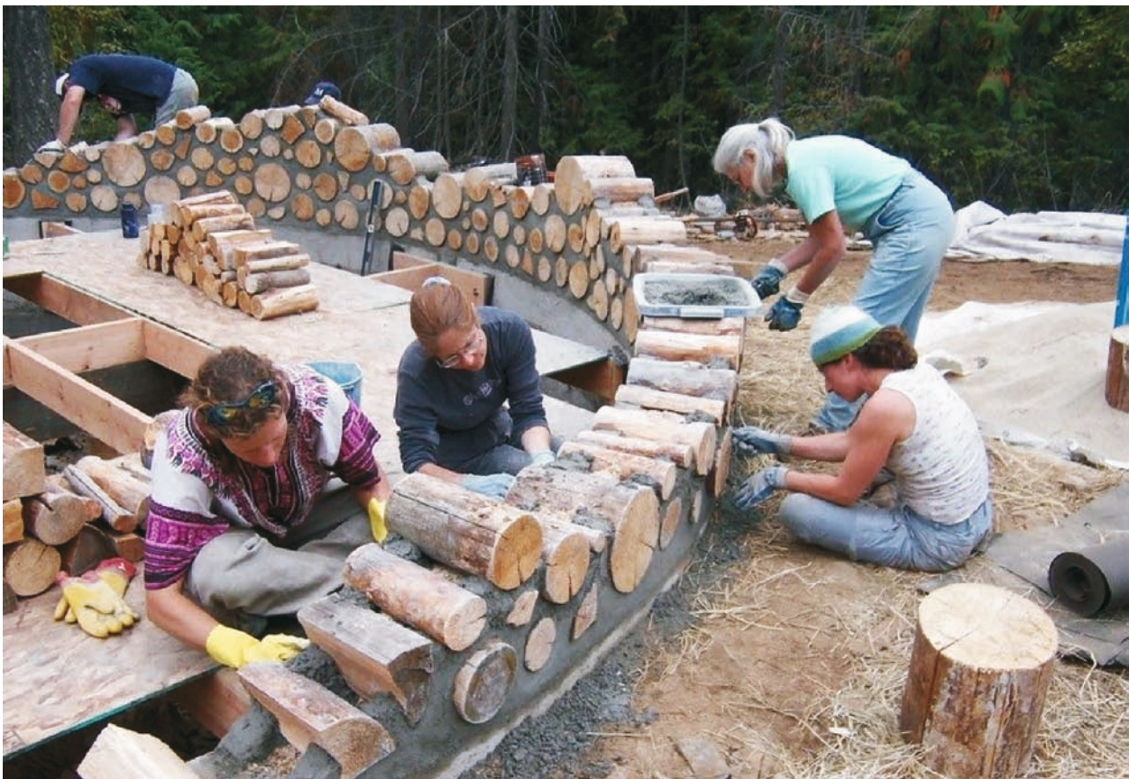
Fig. 1. A cordwood masonry construction site; photo by: [Roy, 2017]
