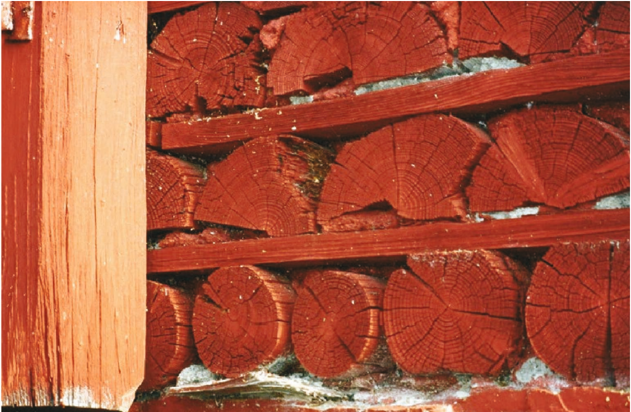
Fig. 23. A closeup of the wall seen in Fig. 22. There is for the most part wood resting on wood, so there is continuous vertical wood on wood contact. In this case the wood can be said to be load bearing for the most part alone [SINTEF Byggforsk, 2017, p. 3].
