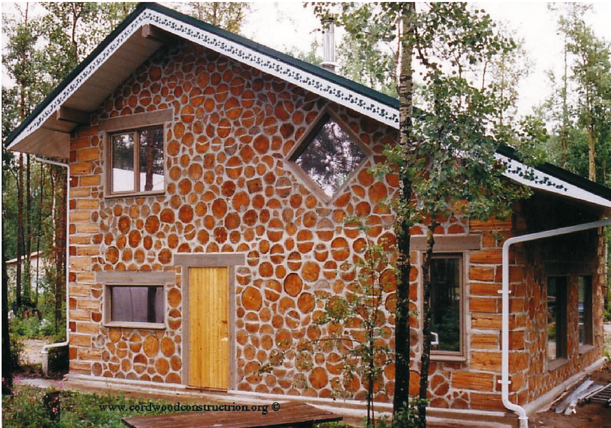
Fig. 4. Newer cordwood house in North America; photo by: [Flatau, n.d.b]
