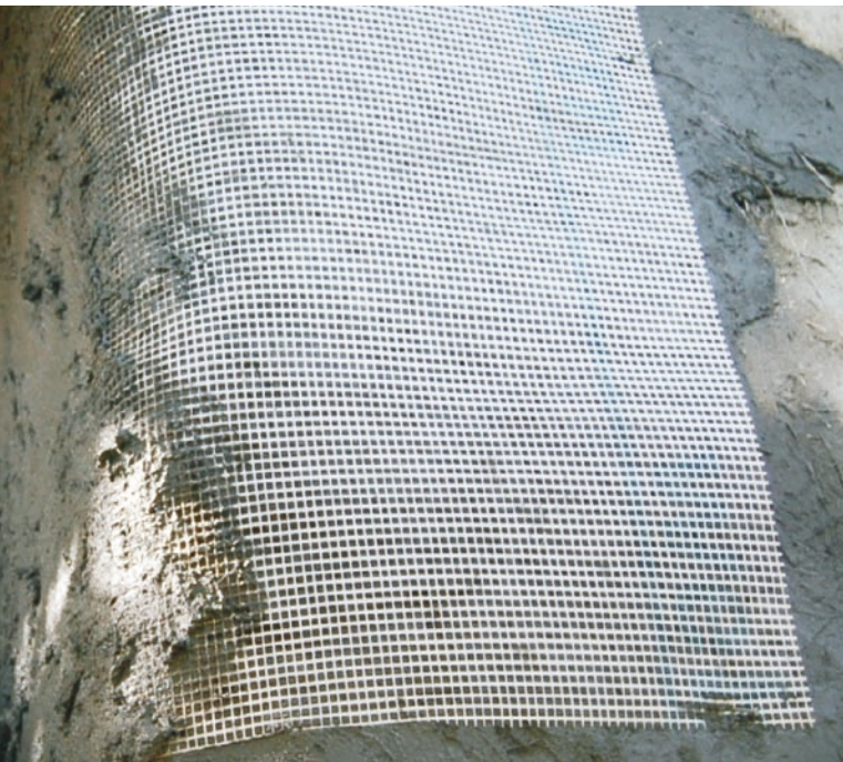
Fig. 33. Photo from straw bale house. Glass fiber mesh on first layer to give adherence to the next layer, 2015; photo by the author
