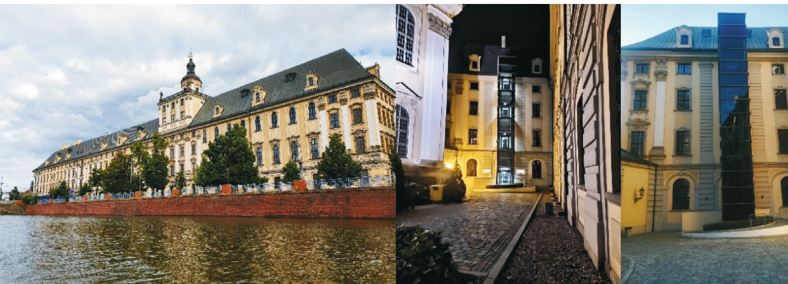
Fig. 10. University of Wrocław – exterior lift; source: photo by the authors
