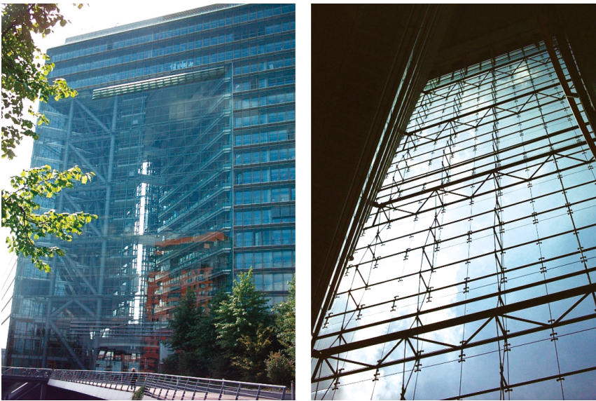
FIG. 6.16. Example of suspended glazing. Note the vertical bracing in the photo. Stadttor, Düsseldorf – Germany. Designer: Petzinka Pink und Partner (Source: photos by V. Di Naso)
