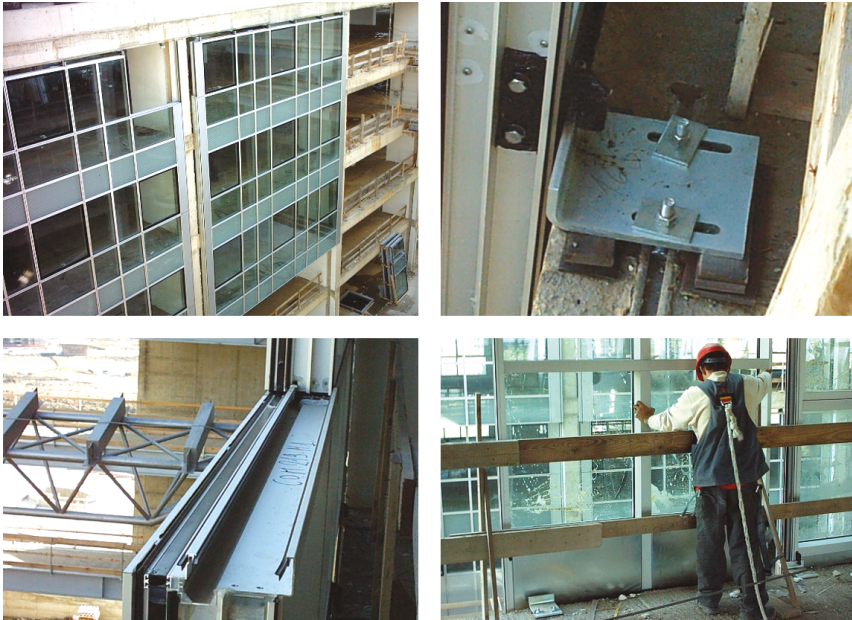
FIG. 6.10. View of the facade under construction (top left), a fixing bracket detail (top right), detail of the upper “half transom” of a module of a unitised curtain wall module (bottom left) and assembly phase of a unitised curtain wall module (bottom right). New Palace of Justice in Florence – Italy. Designer: Arch. Leonardo Ricci (Source: photos by V. Di Naso)
