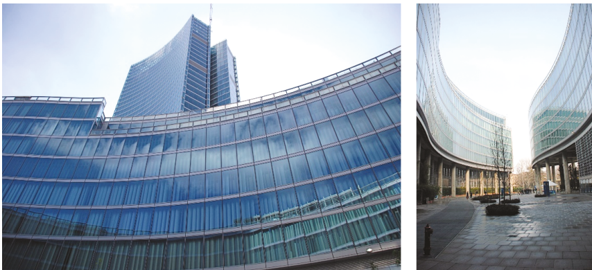
FIG. 6.6. Example of unitised curtain wall. Region Lombardy Headquarters in Milano – Italy. Designer: Pei Cobb Freed & Partners (Source: © courtesy of METRA Spa)
