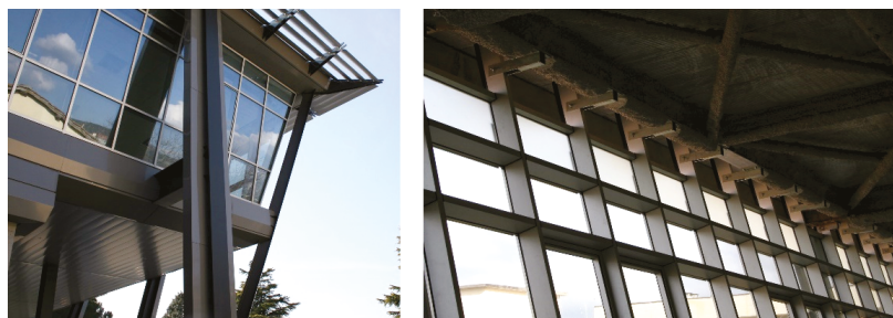
FIG. 6.2. Example of stick system façades with mechanical fixing. Expansion of El.En. S.p.A. factory, Calenzano (FI) – Italy. Designer: Vincenzo Di Naso (Source: photos by V. Di Naso)
