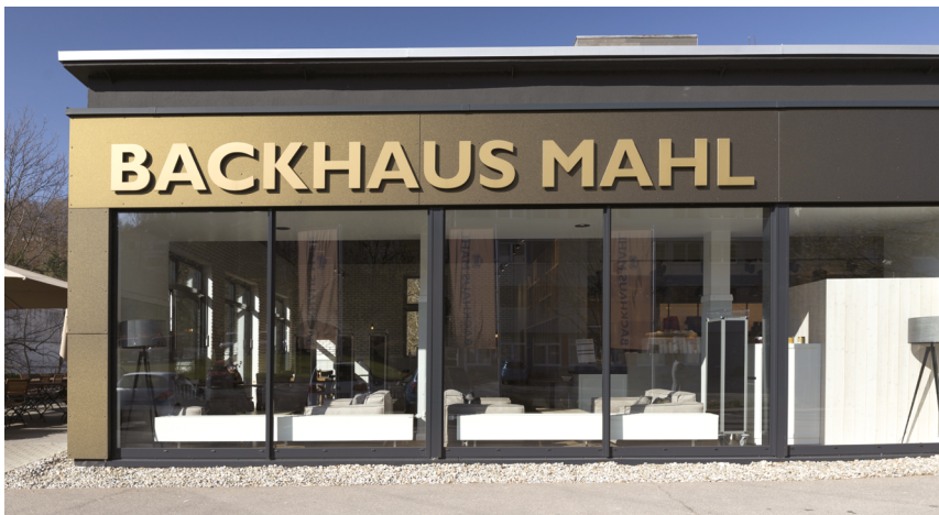
FIG. 5.8. Point fixing system through the cladding, with mullions. Backhaus Muhl, Albstadt-Tailfingen – Germany (Source: © Courtesy of Alucobond, © Elisabeth Leblanc)
