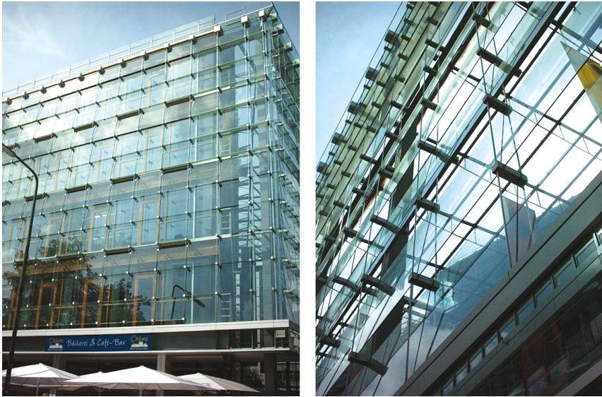
FIG. 6.15. Example of point-fixed glass façade with clamp. Office building H19, Düsseldorf – Germany. Designer: Petzinka Pink und Partner (Source: photos by V. Di Naso)
