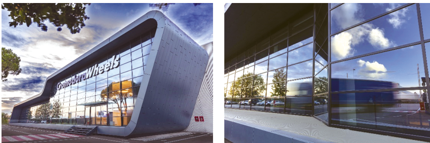
FIG. 6.5. Example of site-assembled traditional stick system façades. Commodora Wheels building in Ghedi (BS)– Italy. Designer: Studio Associato di Ingegneria Civile Ingg. Vecchi (Source: © courtesy of METRA Spa)
