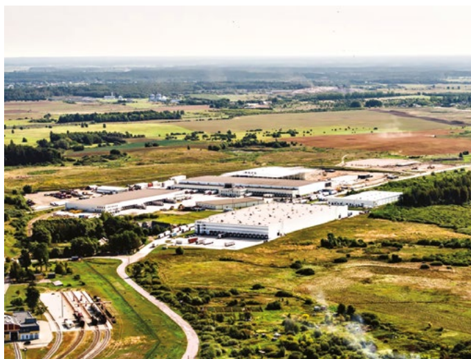
FIG. 8.2. Picture BLC logistics center (Source: own elaboration, 2019)
