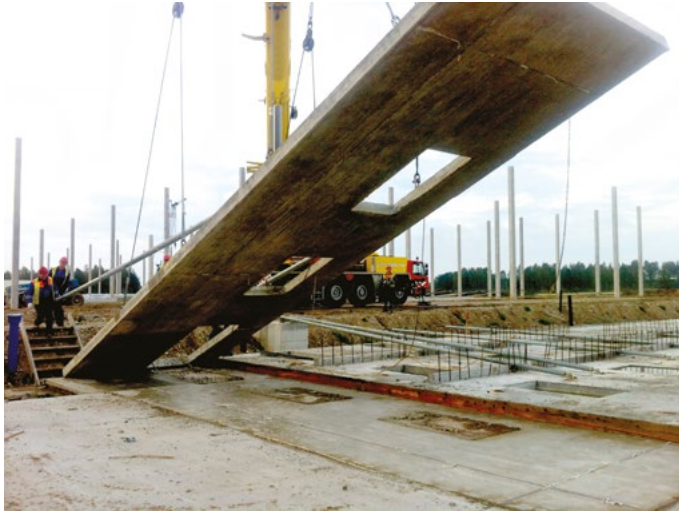
FIG. 8.2. Tilt-up panel (Source: own elaboration, 2018)
